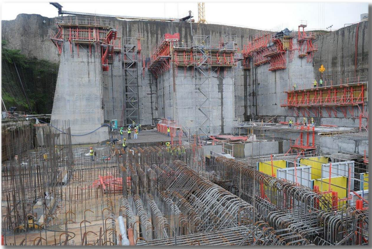
Fig. 1 – Massive concrete blocks of New Panama Canal
