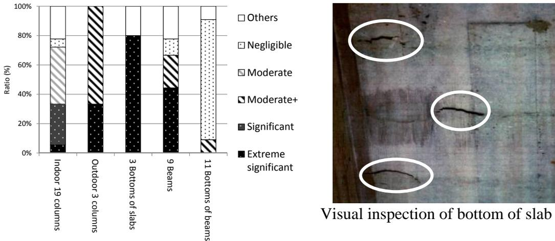
Figure 11: Rate of steel bar corrosion in NMWA
